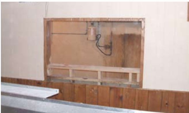
The new framing to bring it up to the correct height.
